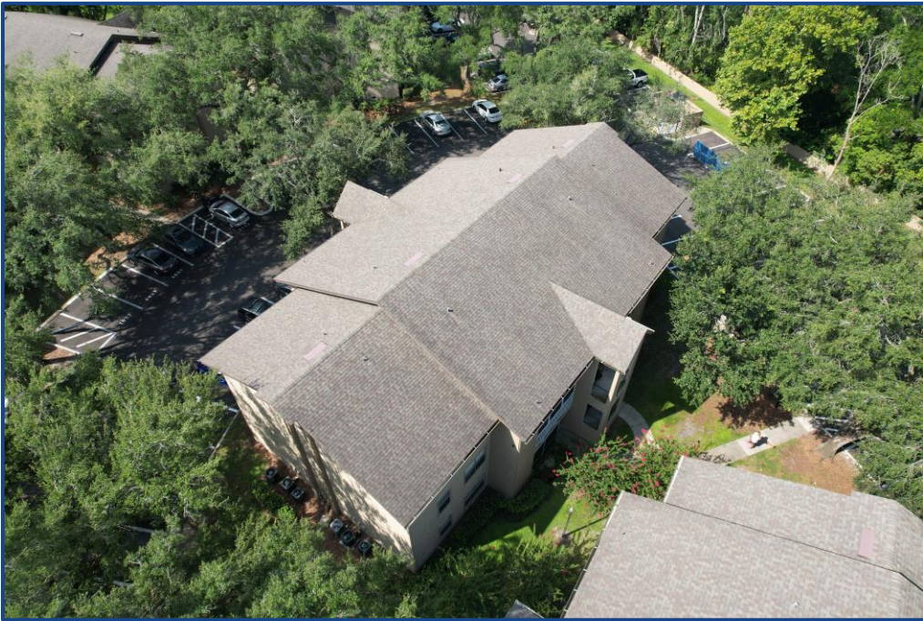
Photograph No. 4: North elevation.
