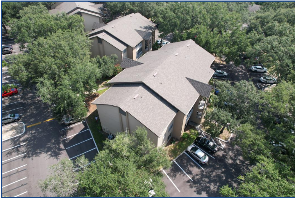
Photograph No. 2: South elevation.
