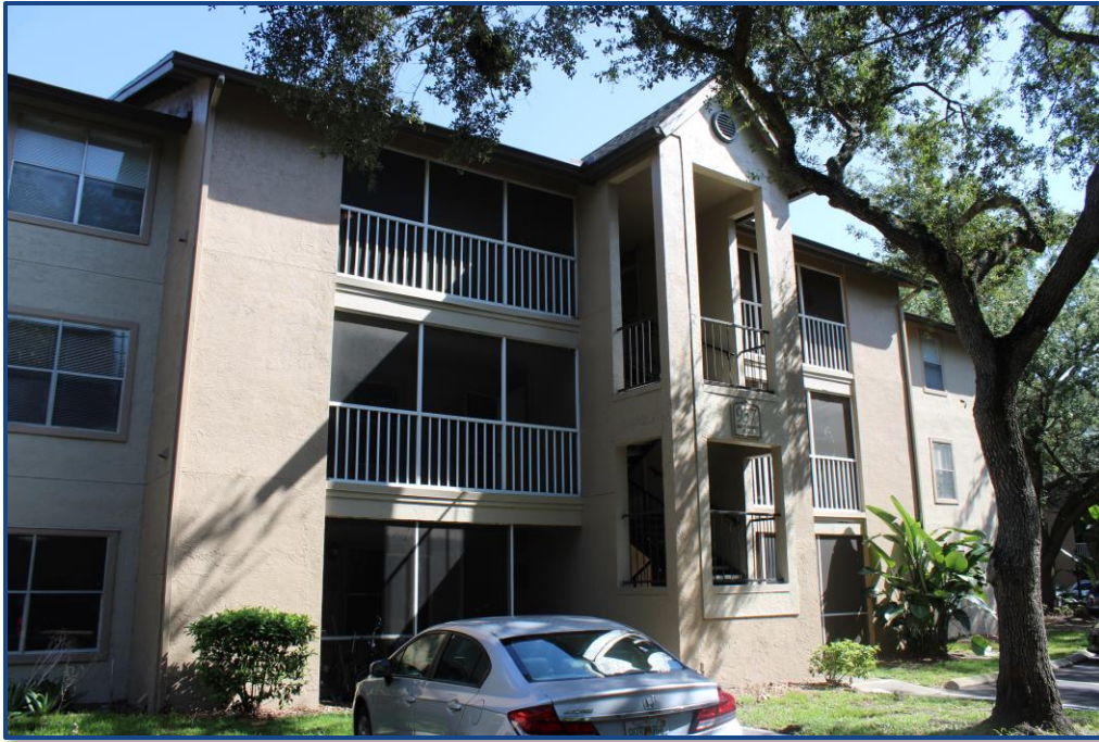
Photograph No. 9: View of the balconies and stairway on the south side of the building.
