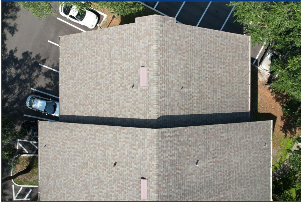
Photograph No. 5: View of the west roof section.
