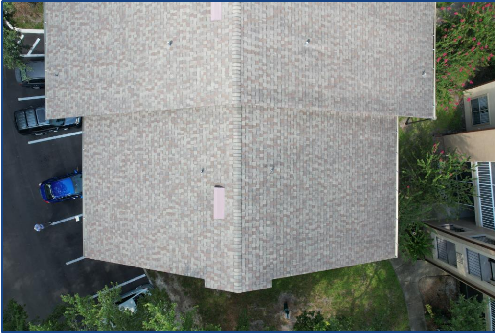
Photograph No. 7: View of the east roof section.
