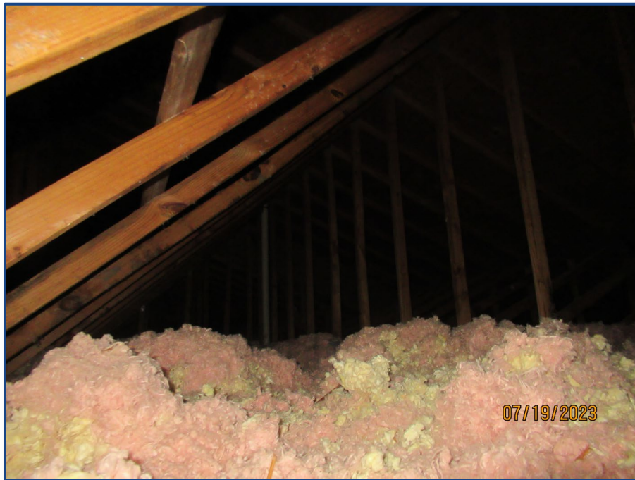
Photograph No. 8: General view of the prefabricated wooden roof trusses.
