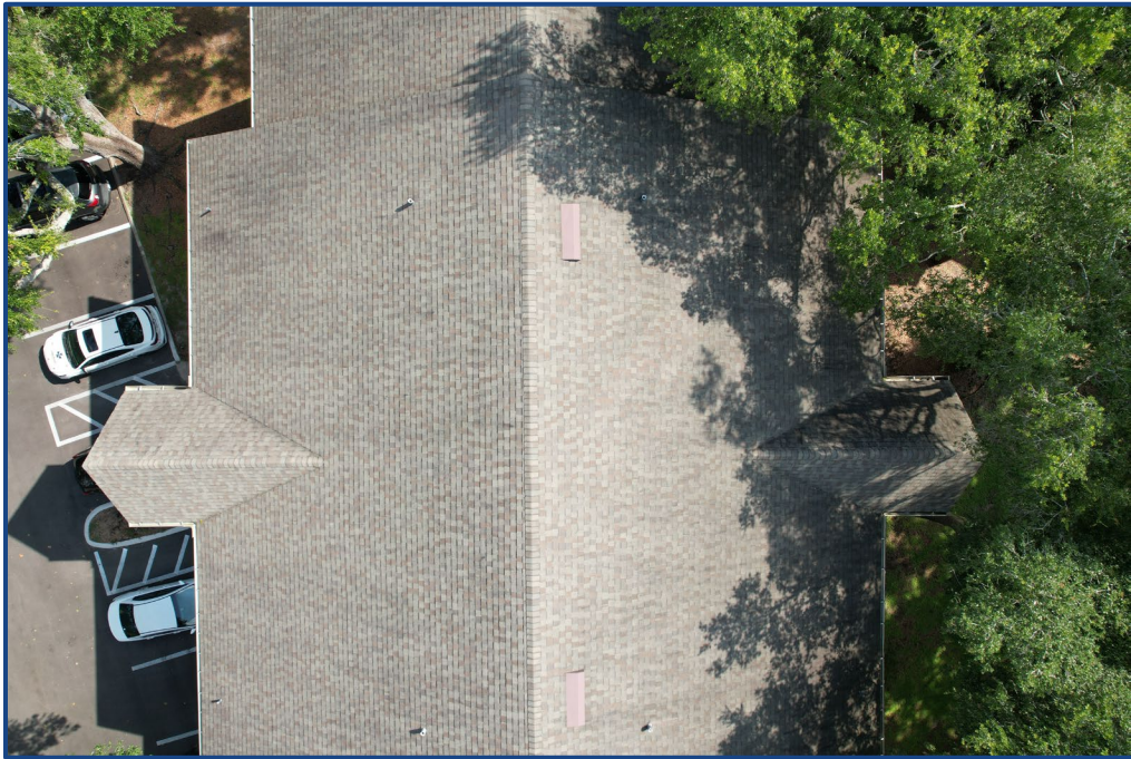
Photograph No. 6: View of the central roof section.
