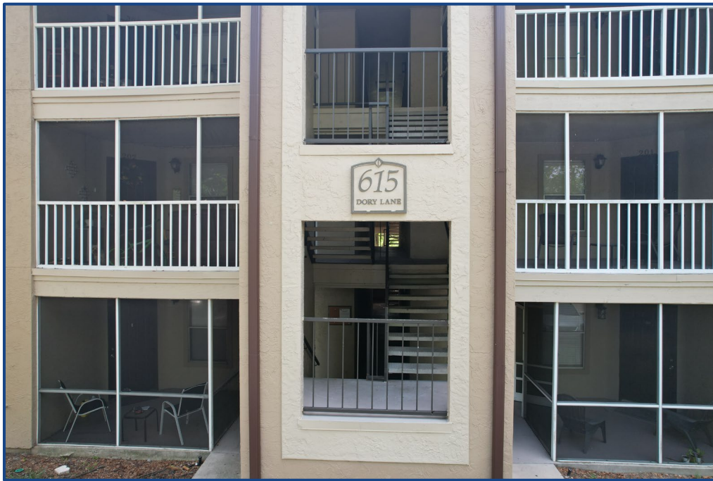
Photograph No. 10: View of the balconies and stairway on the west side of the building.
