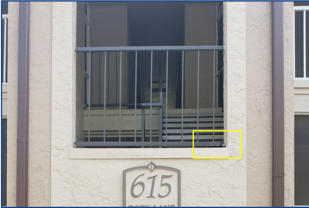
Photograph No. 19: Corrosion to the metal guardrail located in the west stairway.
