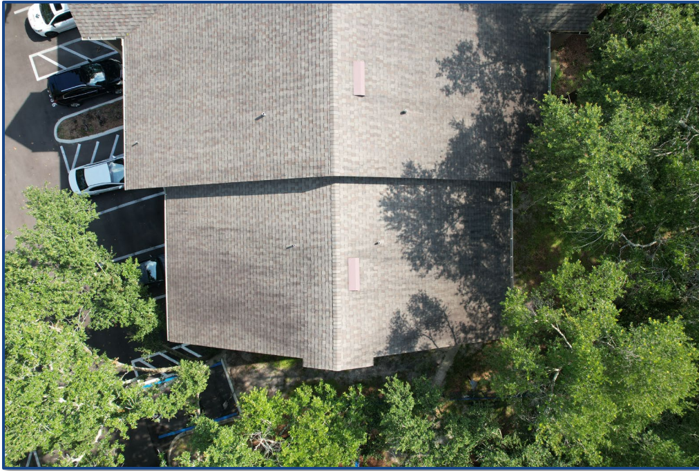
Photograph No. 7: View of the south roof section.
