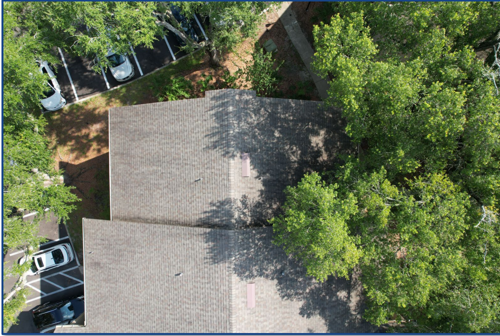
Photograph No. 5: View of the north roof section.
