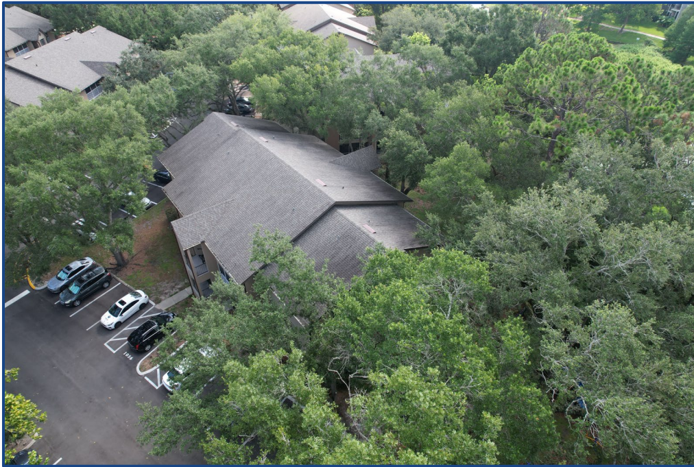
Photograph No. 2: West elevation.
