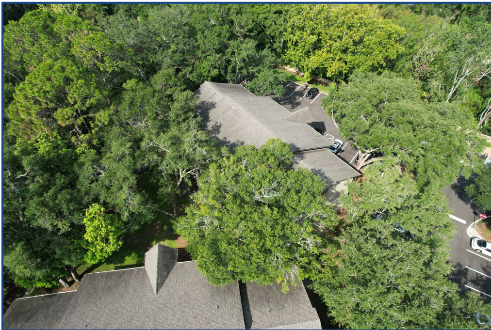
Photograph No. 4: East elevation.
