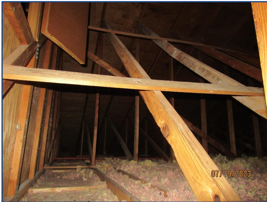
Photograph No. 6: General view of the prefabricated wooden roof trusses.
