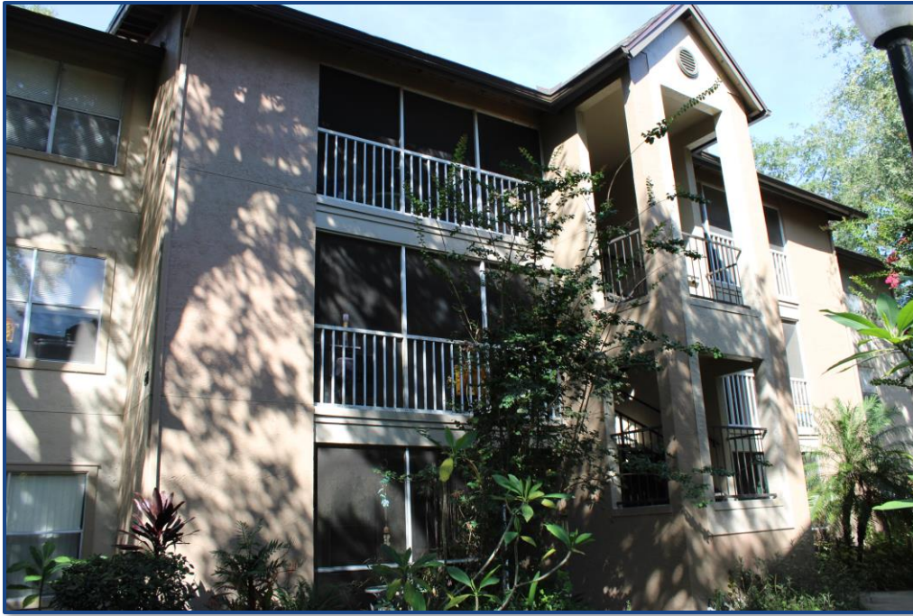
Photograph No. 7: View of the balconies and stairway on the east side of the building.
