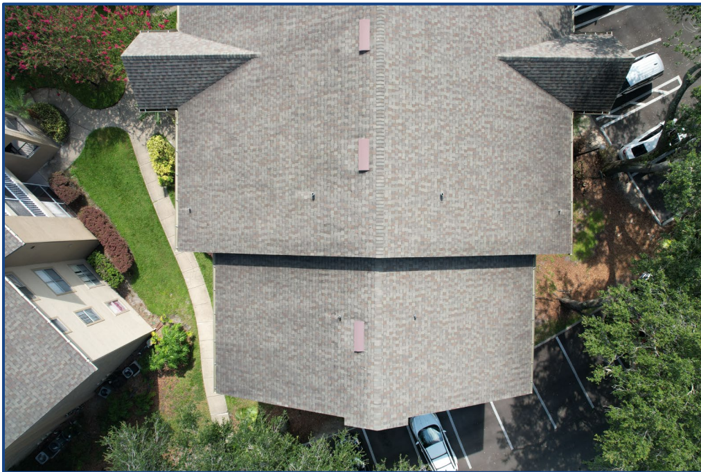
Photograph No. 6: View of the west roof section.
