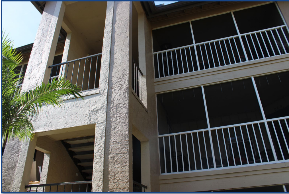
Photograph No. 9: View of the balconies and stairway on the north side of the building.
