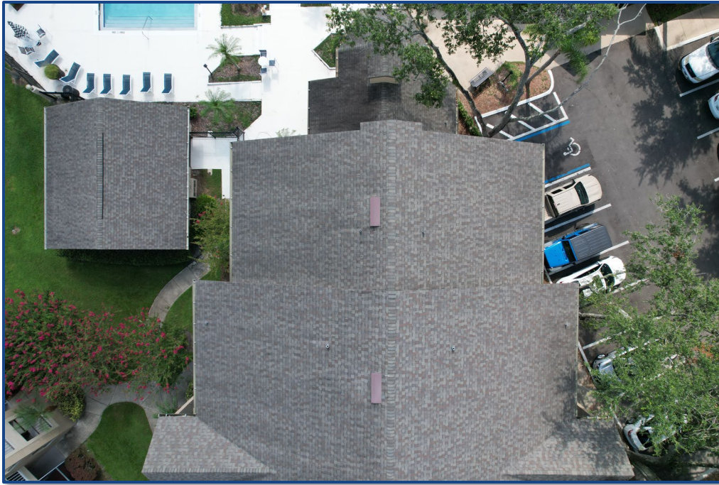
Photograph No. 5: View of the east roof section.
