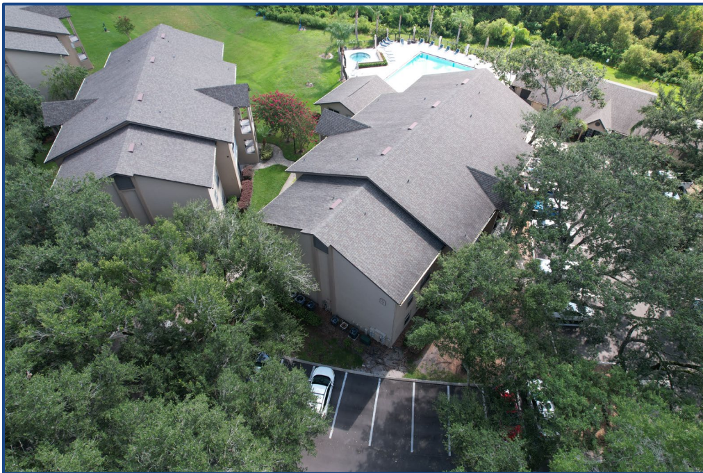
Photograph No. 4: West elevation.
