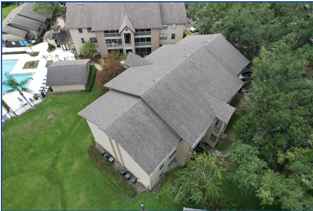
Photograph No. 4: North elevation.
