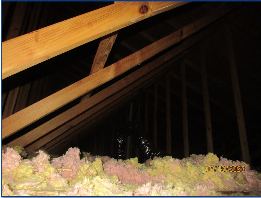
Photograph No. 7: General view of the prefabricated wooden roof trusses.
