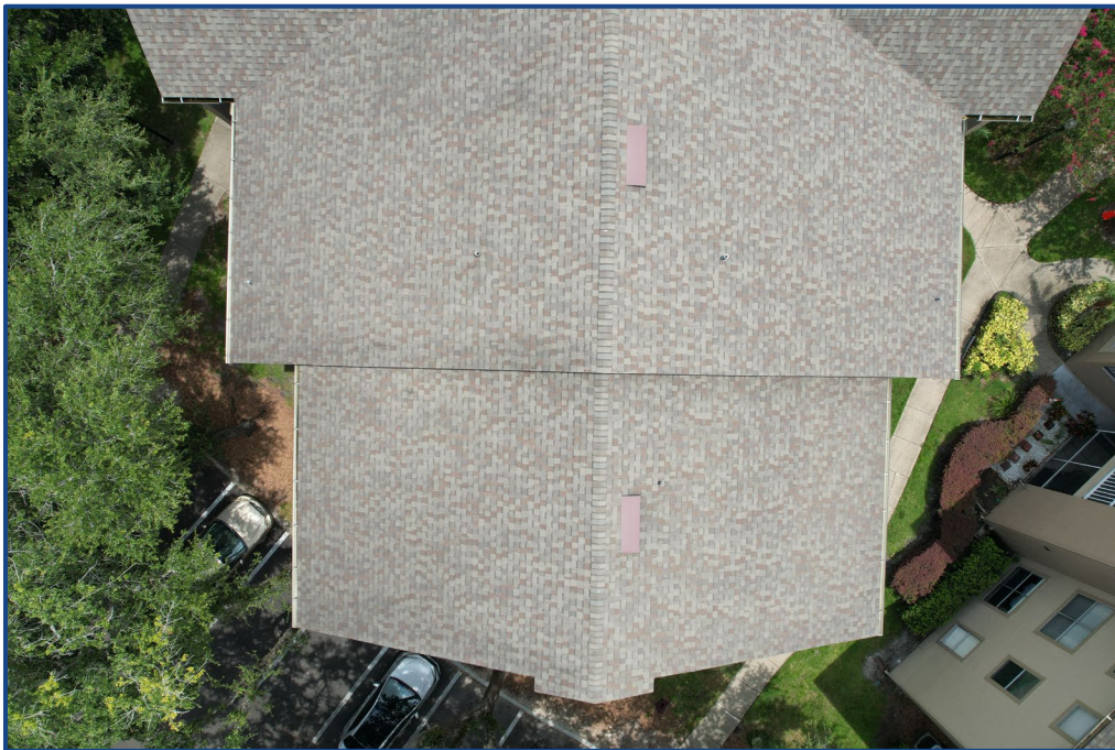
Photograph No. 6: Overview of the southwest roof section.
