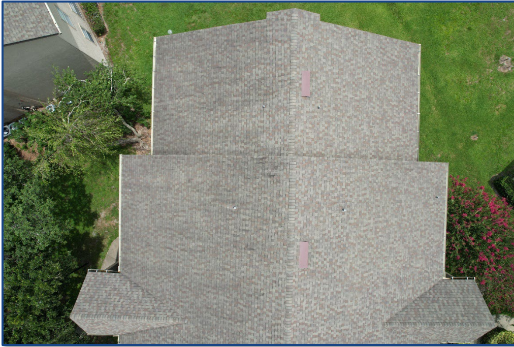
Photograph No. 5: Overview of the northeast roof section
