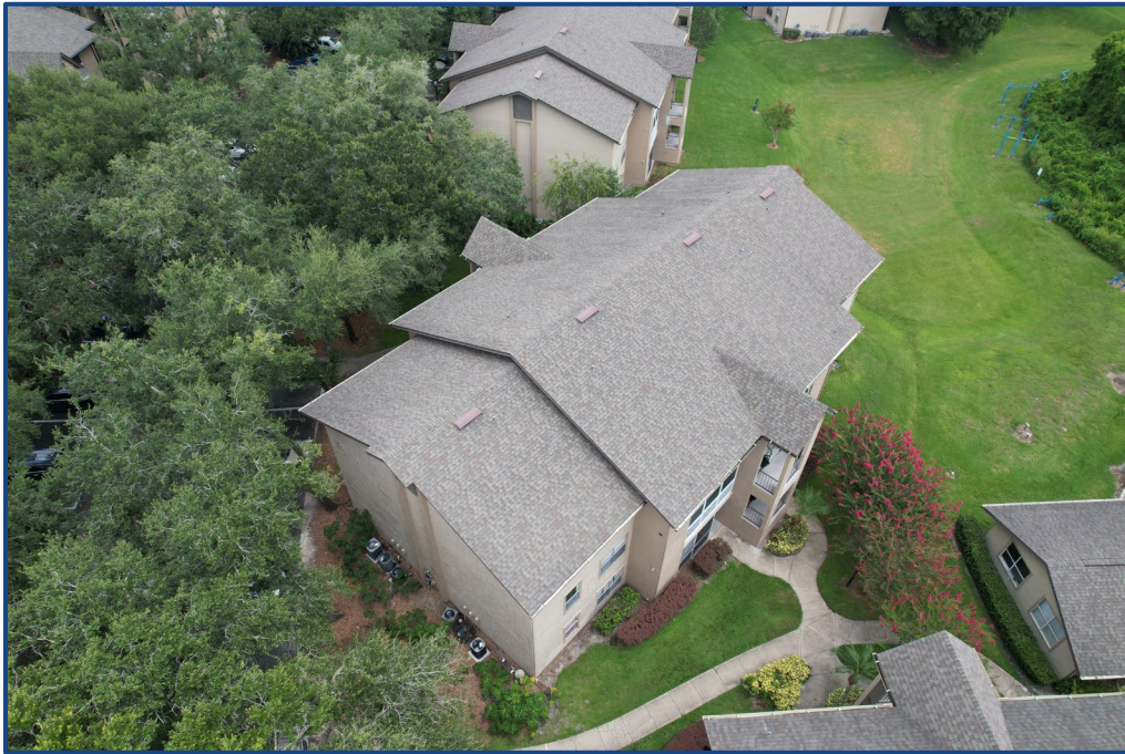
Photograph No. 2: South elevation.
