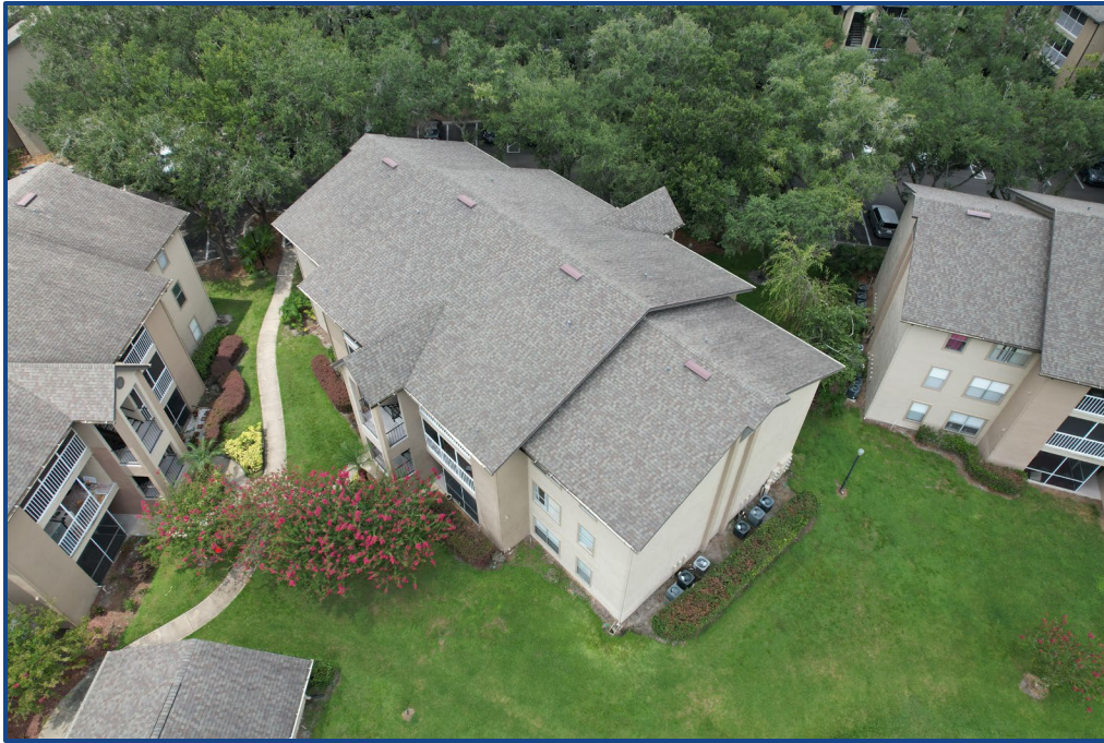
Photograph No. 3: East elevation.
