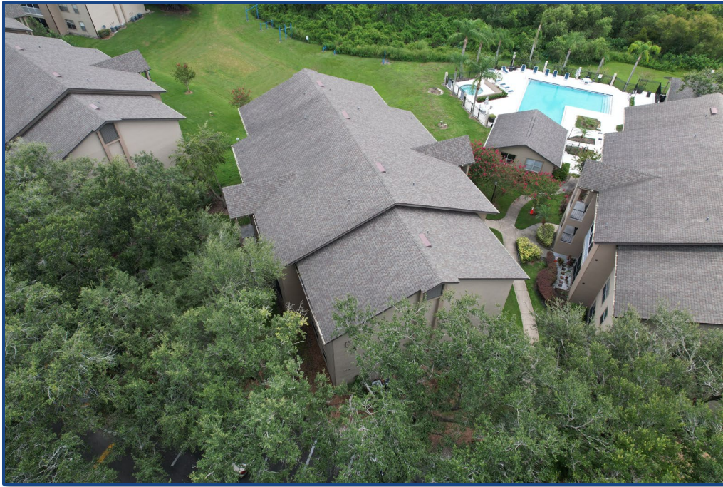
Photograph No. 1: West elevation.
