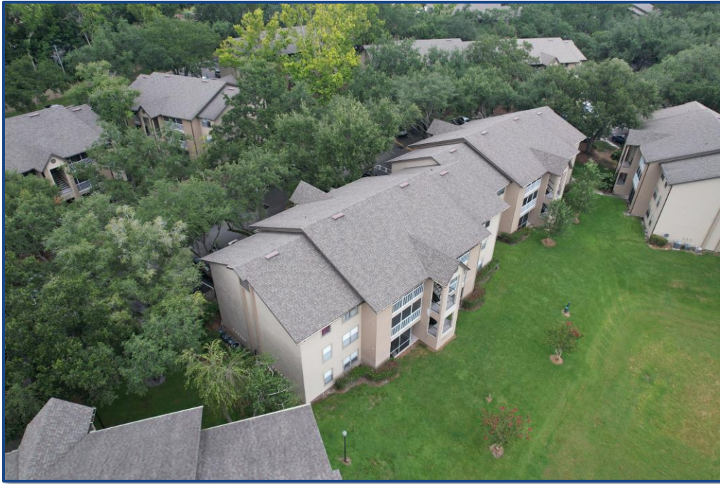
Photograph No. 3: South elevation.
