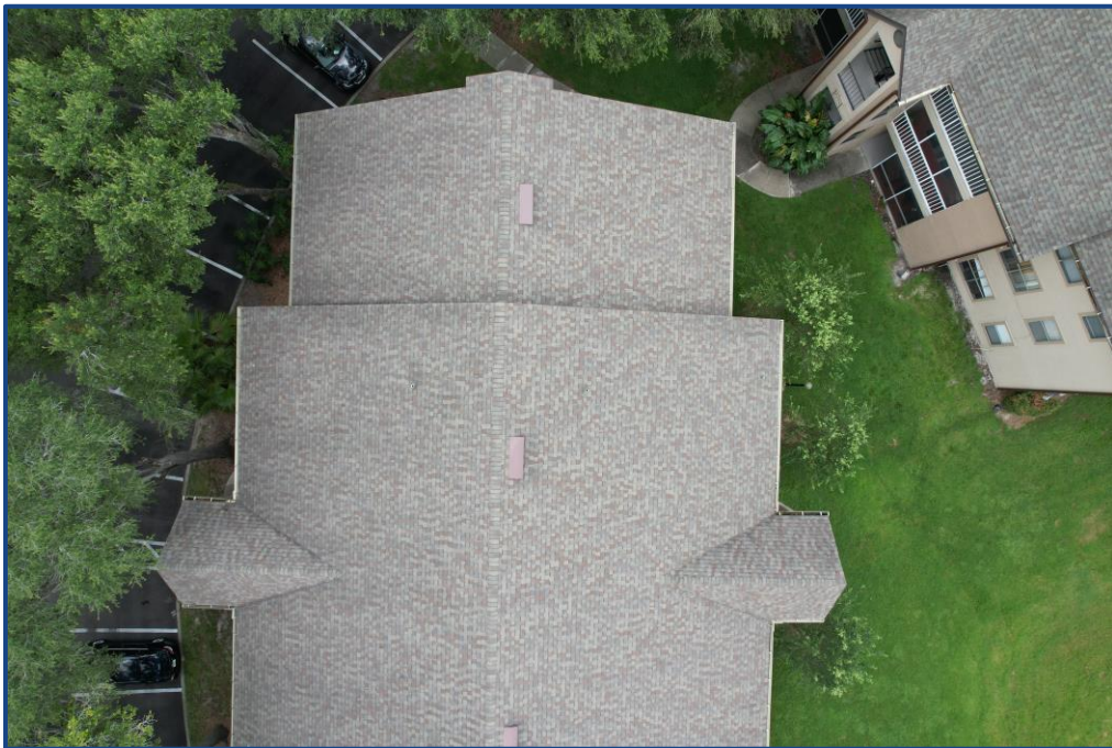
Photograph No. 8: View of the north roof section.
