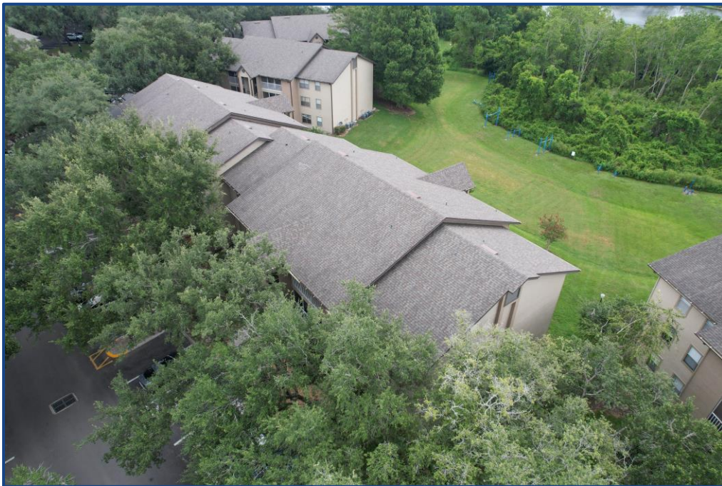
Photograph No. 2: West elevation.
