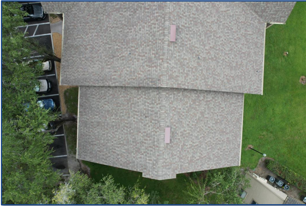
Photograph No. 5: View of the south roof section.
