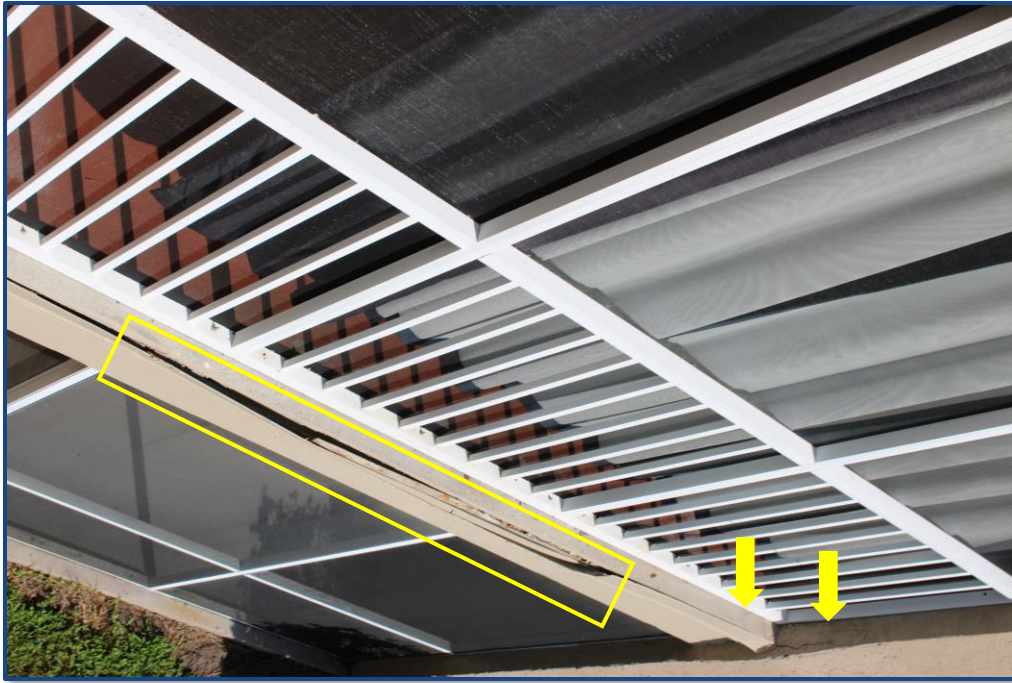
Photograph No. 15: Cracks in the stucco wall finish, crack in the balcony slab, and damage to the metal flashing at the edge of the balcony slab on Unit 207.
