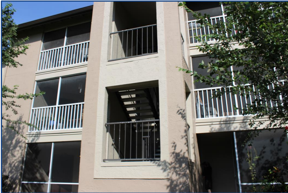
Photograph No. 10: View of the balconies and stairway on the northeast side of the building.
