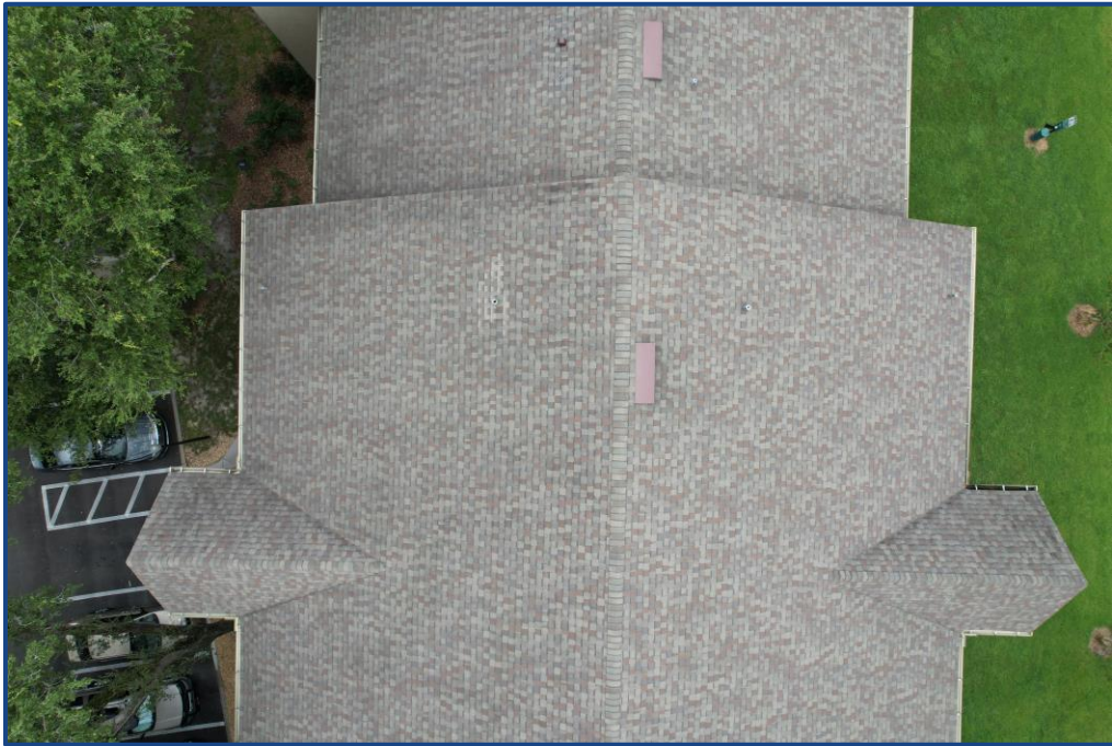
Photograph No. 6: View of the south roof section.
