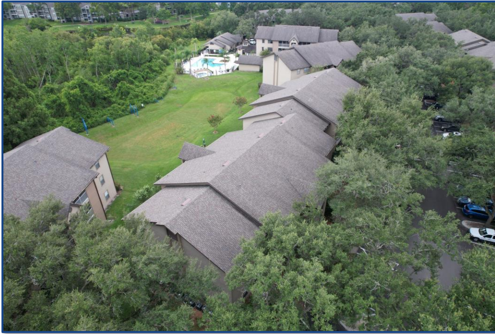
Photograph No. 1: North elevation.
