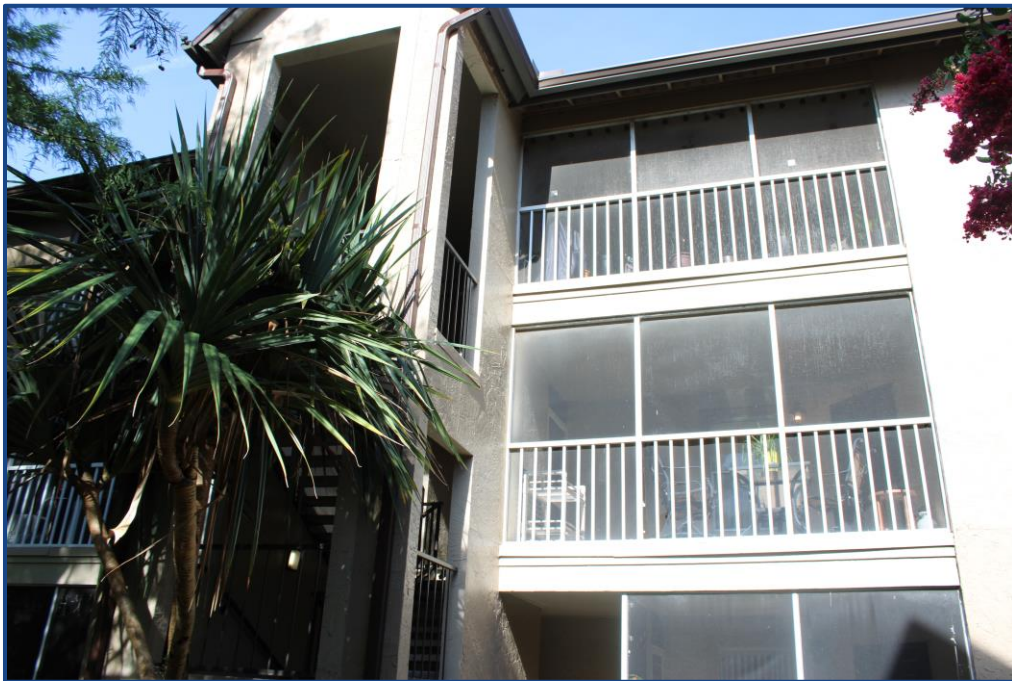
Photograph No. 8: View of the balconies and stairway on the east side of the building.
