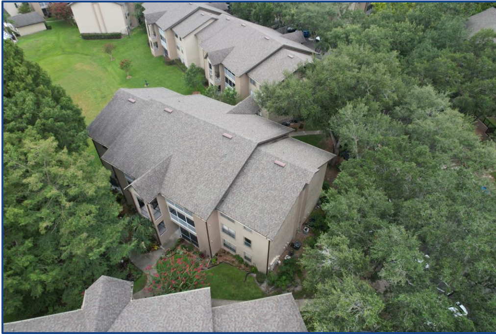
Photograph No. 1: East elevation.
