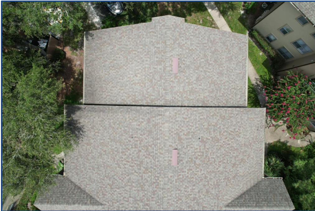
Photograph No. 4: Overview of the north roof section.
