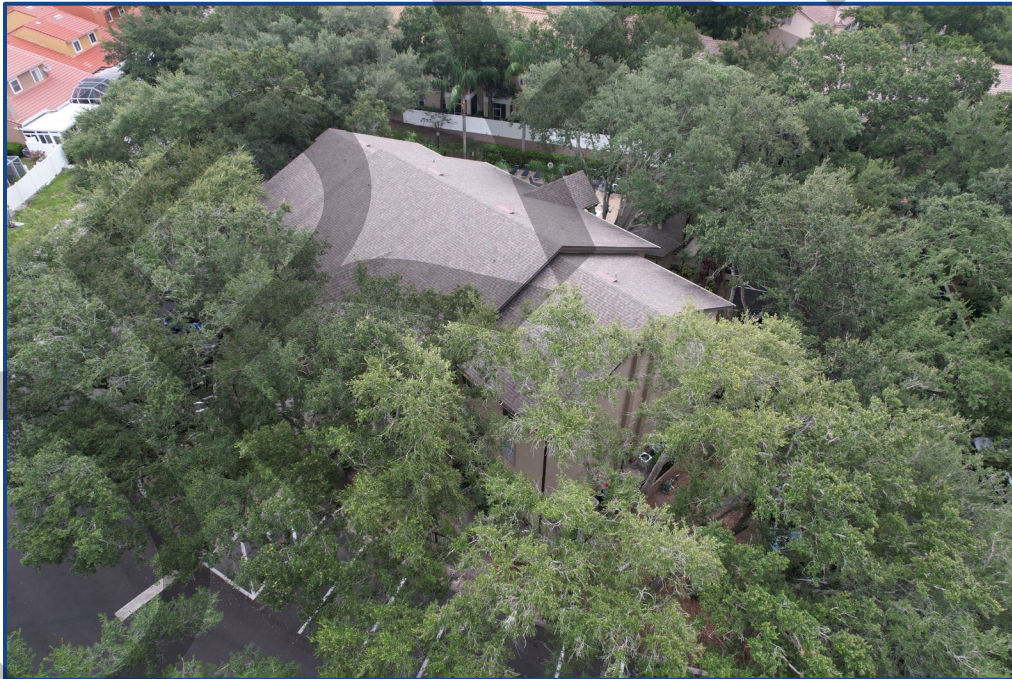
Photograph No. 4: West elevation.
