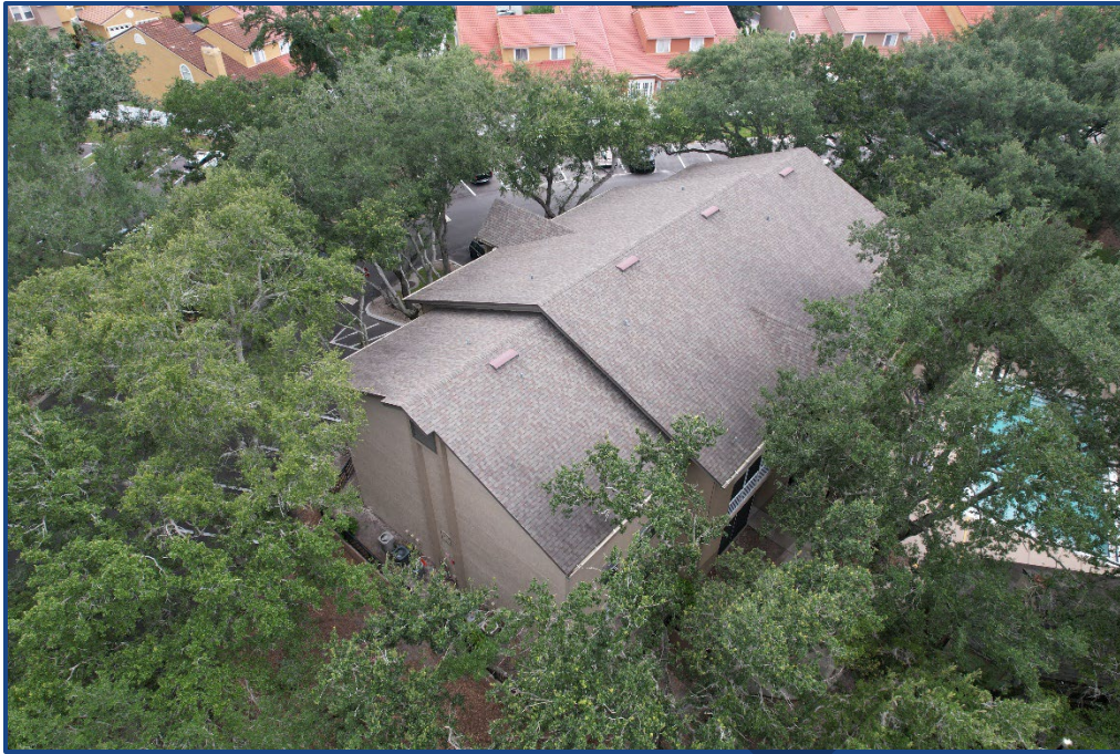
Photograph No. 1: South elevation.
