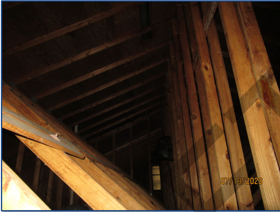
Photograph No. 7: General view of the prefabricated wooden trusses.
