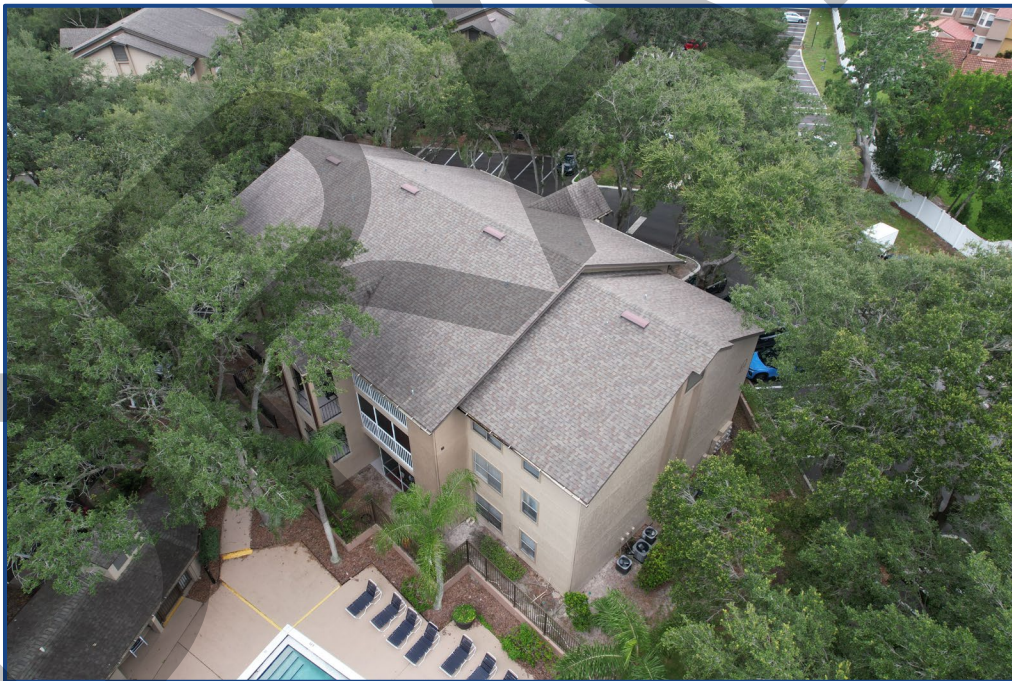
Photograph No. 2: East elevation.
