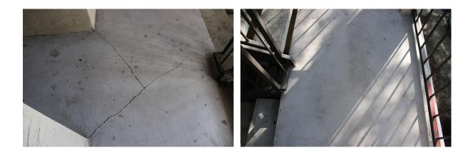
Concrete and Stairway Repairs for year 2024 shall include repairs to cracked cocnrete and corrosion to the steel framing referenced within this report.
