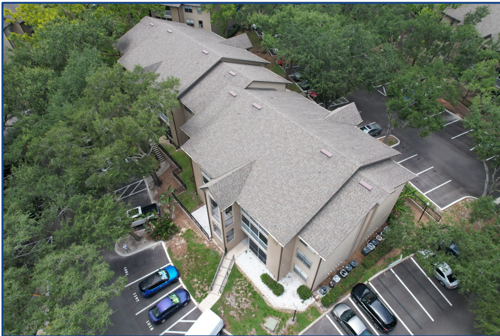
Photograph No. 2: East elevation.
