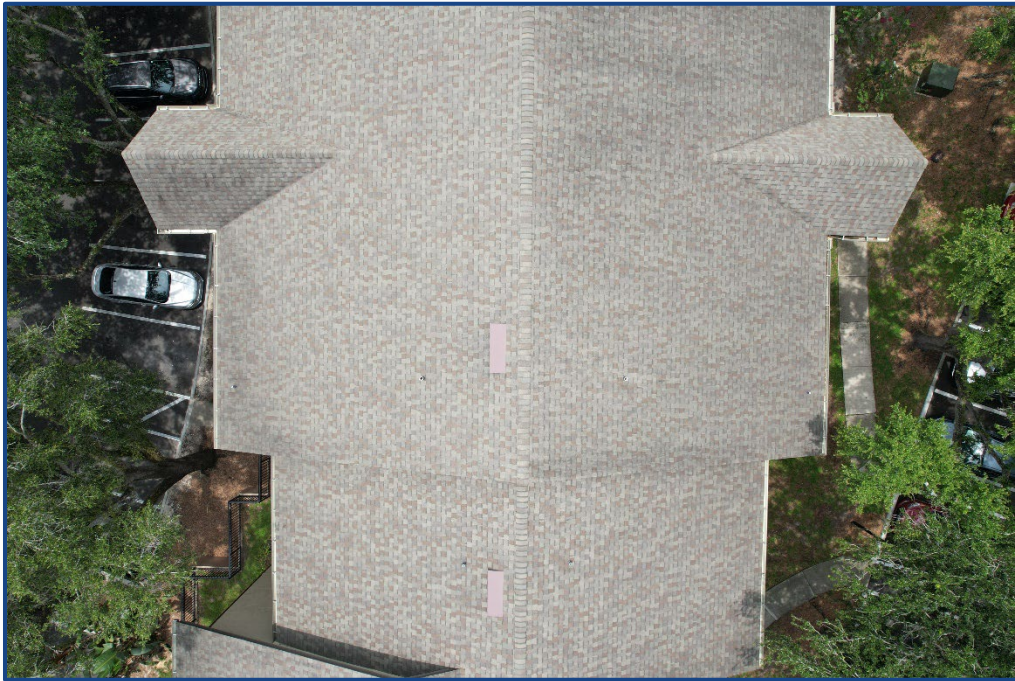
Photograph No. 6: View of the roof.
