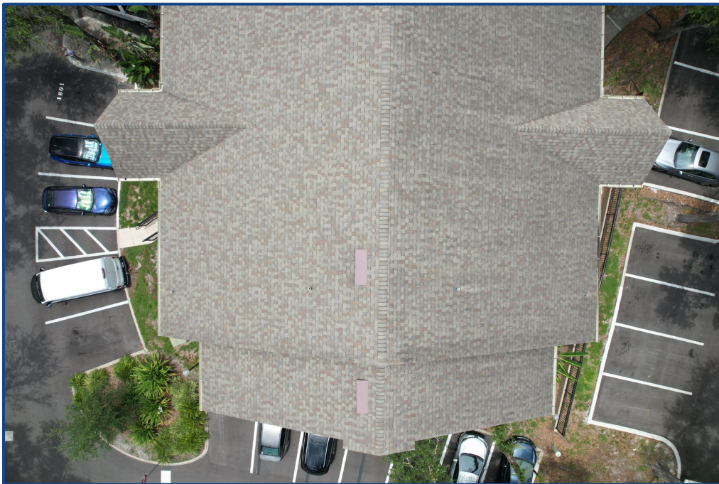
Photograph No. 8: View of the roof.
