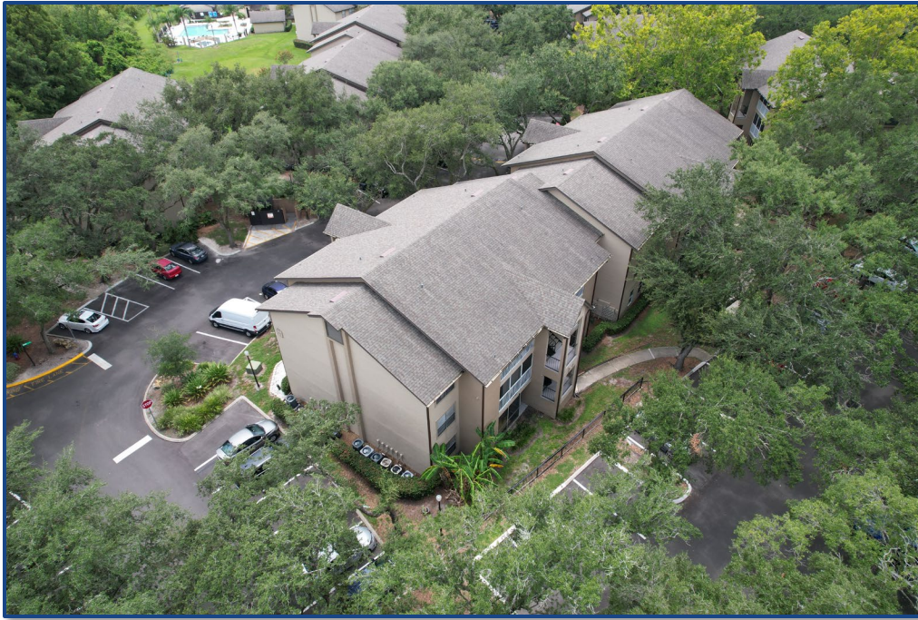
Photograph No. 1: North elevation.
