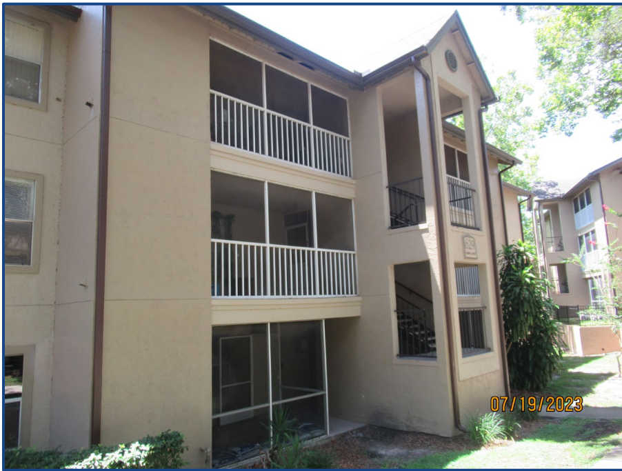
Photograph No. 10: View of the balconies and stairway on the northwest side of the building.
