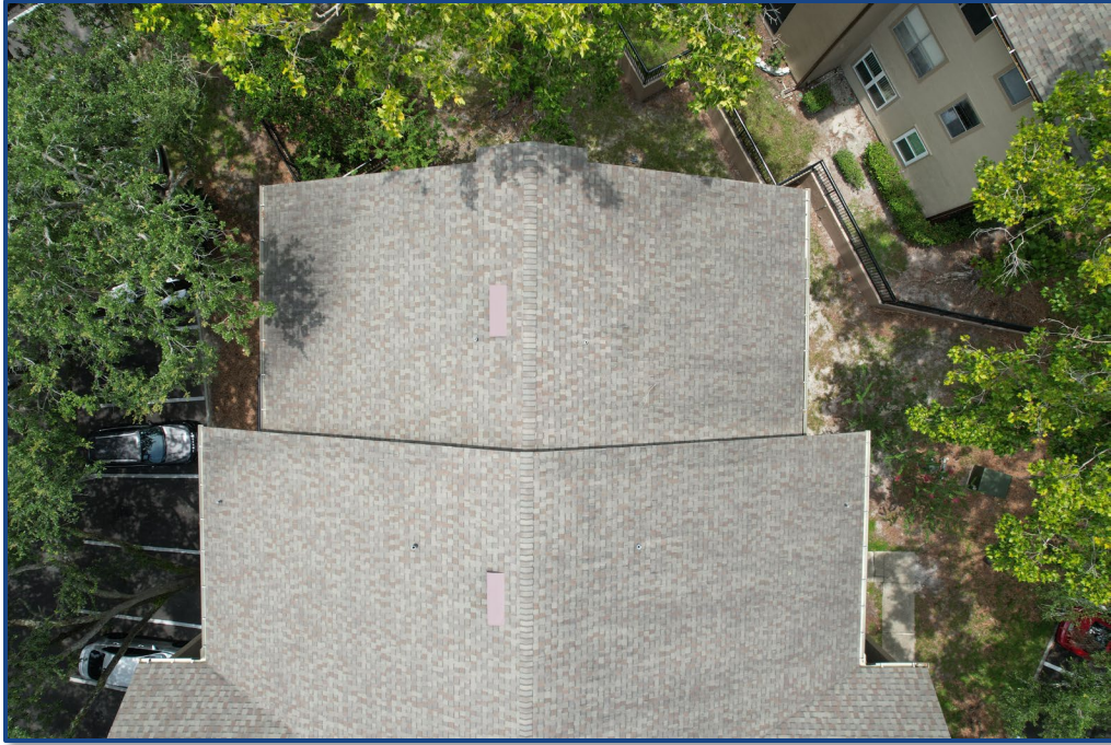
Photograph No. 5: View of the roof.
