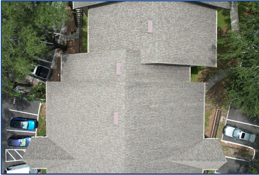
Photograph No. 7: View of the roof.
