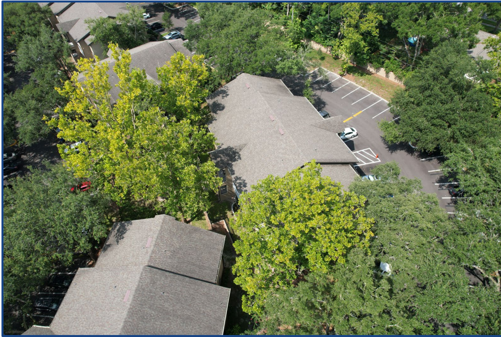
Photograph No. 3: North elevation.
