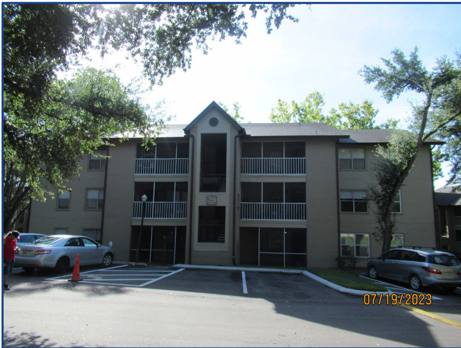
Photograph No. 8: View of the balconies and stairway on the west side of the building.
