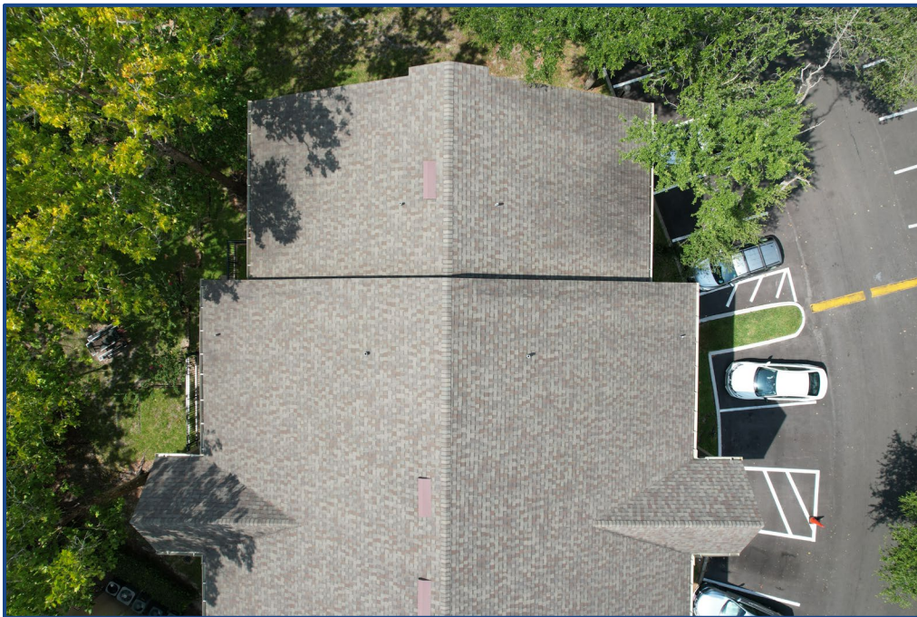
Photograph No. 4: View of the south roof section.
