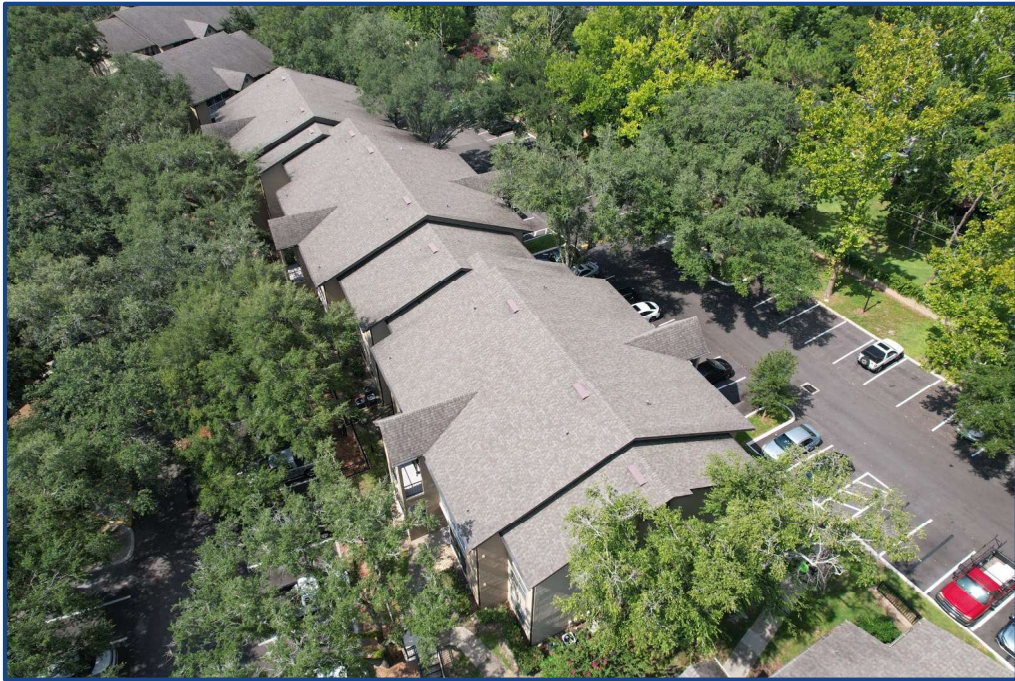
Photograph No. 4: East elevation.
