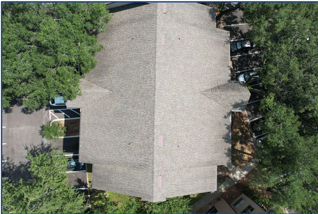
Photograph No. 8: View of the south roof section.
