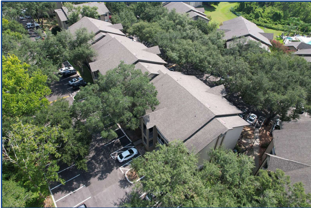
Photograph No. 2: West elevation.
