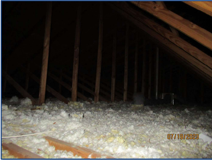
Photograph No. 9: General view of the prefabricated wooden roof trusses.
