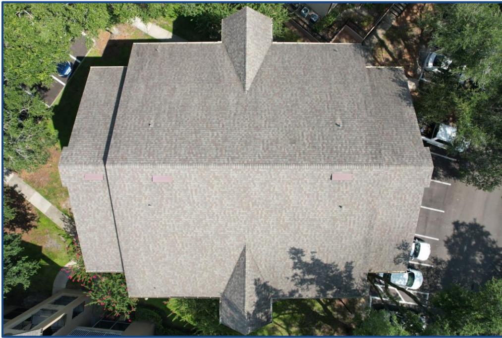
Photograph No. 2: Overview of the roof.
