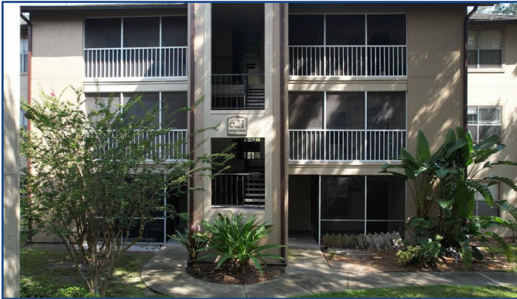
Photograph No. 4: View of the balconies and stairway on the south side of the building.
