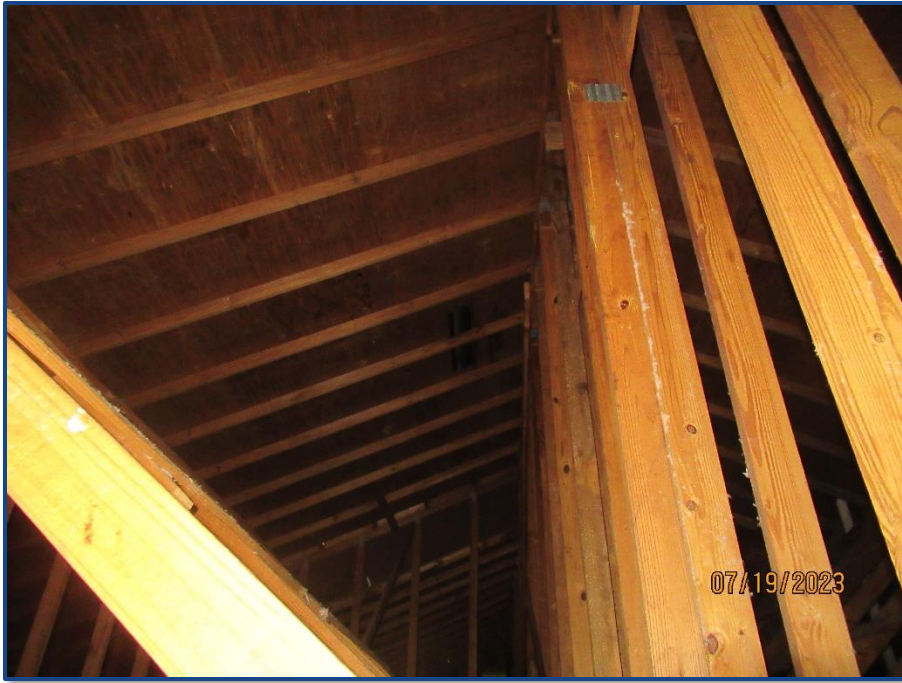
Photograph No. 5: General view of the prefabricated wood roof trusses.
