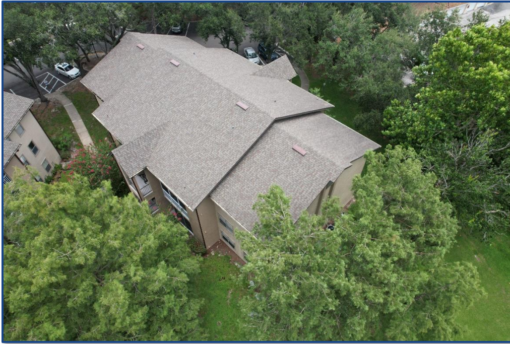
Photograph No. 1: South elevation.
