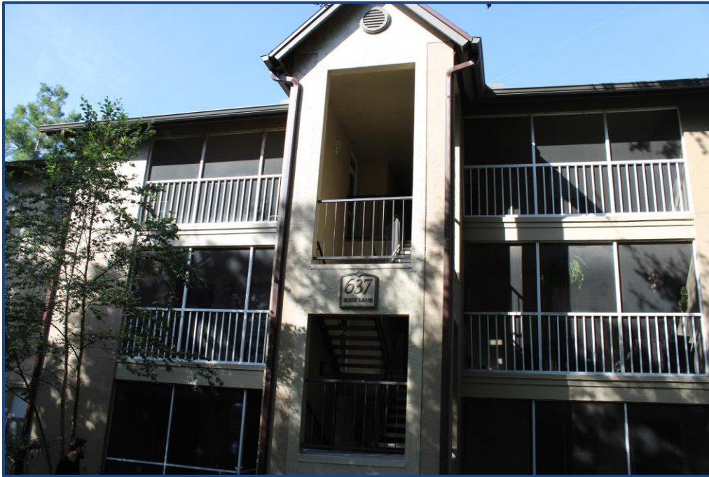
Photograph No. 6: View of the balconies and stairway on the northeast side of the building.
