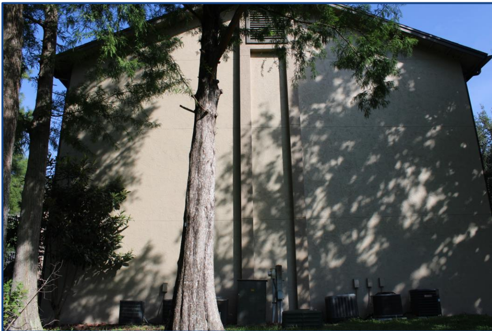
Photograph No. 18: General view of the southeast exterior wall.
