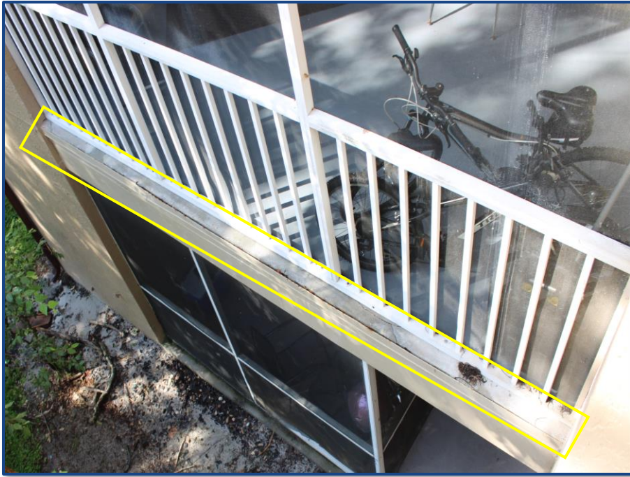
Photograph No. 13: View of cracks in the exterior balcony slab.
