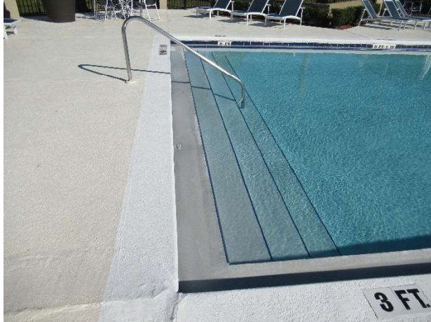
Stair entry, main pool
