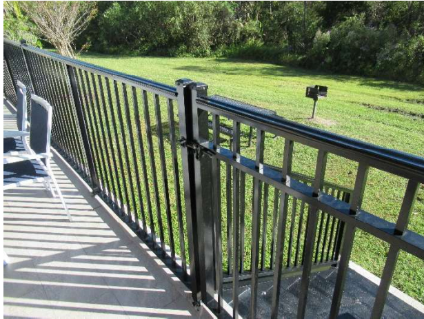
Fence at main pool
