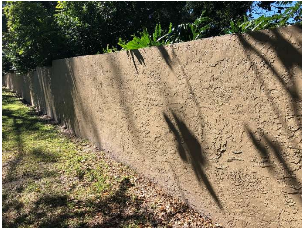
Perimeter wall overview
