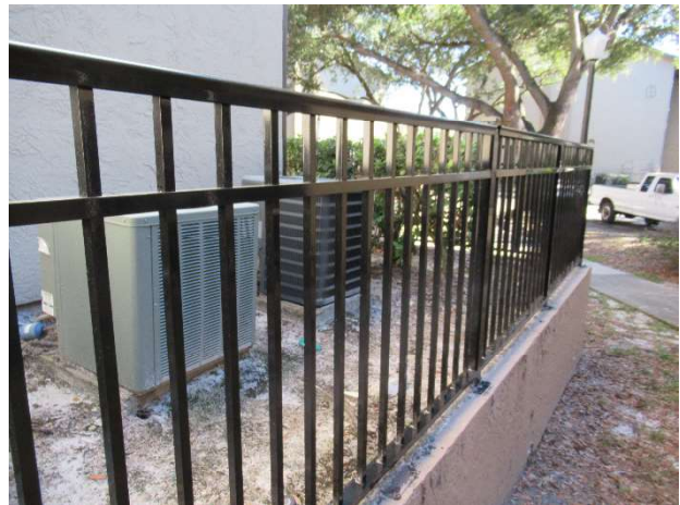
Recently replaced railings
