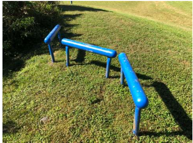
Paint finish deterioration at fitness equipment
