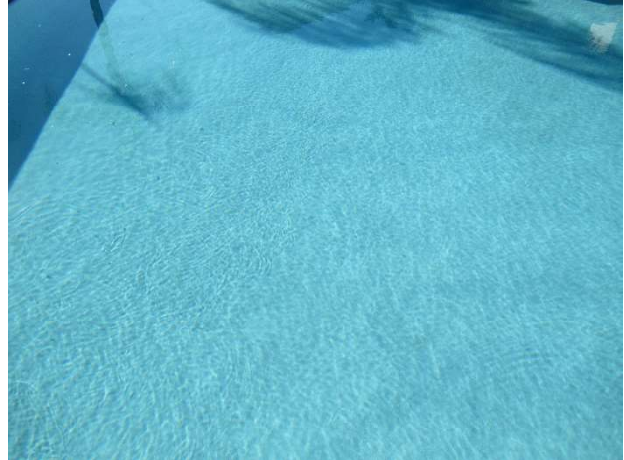
Plaster overview, main pool
