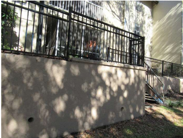
Retaining wall overview
