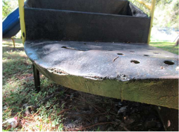
Bent step with rust present
