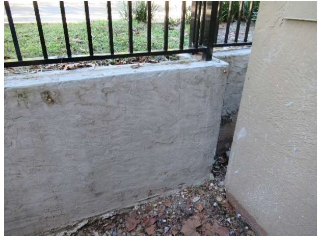
Retaining wall overview (finishes are inconsistent with remainder of community)
