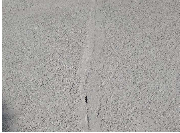
Repairs at main pool deck
