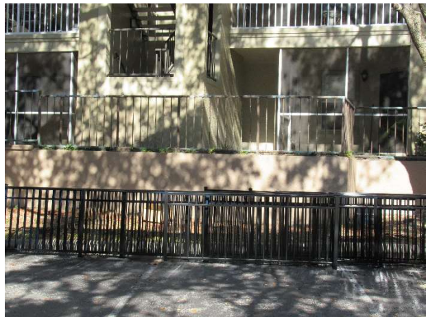
Railings awaiting installation
