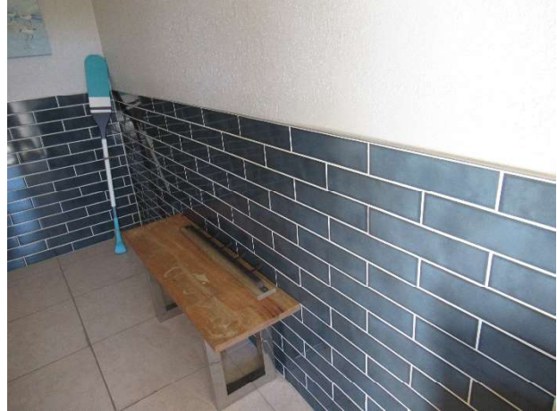
Rest room wall coverings
