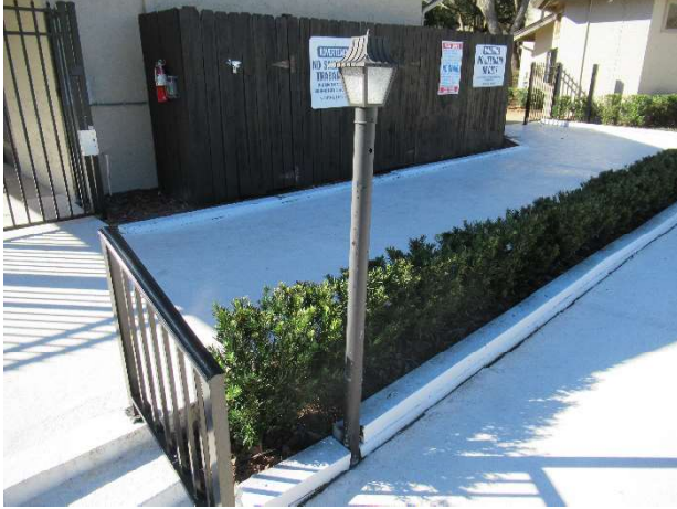
Light pole and fixture
