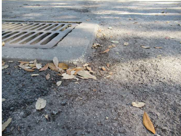
Catch basin crown detail view
