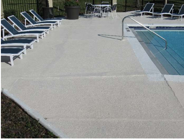
Main pool deck
