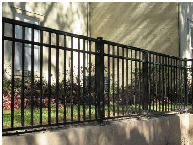
Recently replaced railings
