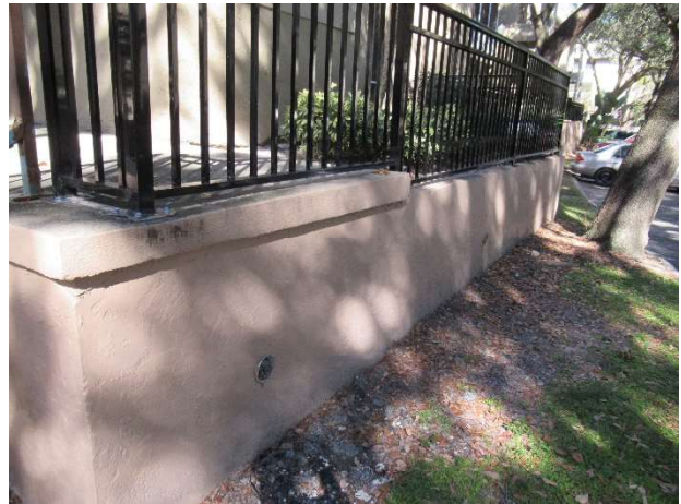
Retaining wall overview
