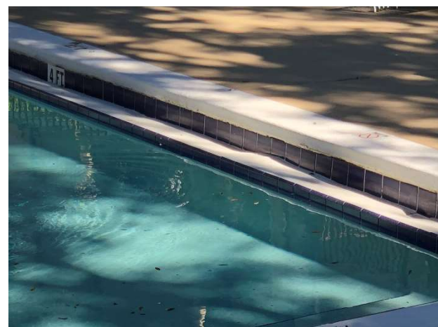
Plaster and tile overview, lap pool
