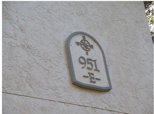
Detail view at building identification signs
