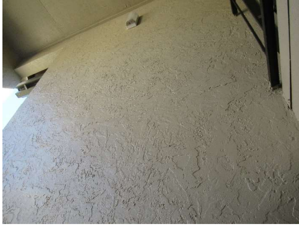
Stucco finishes at staircases
