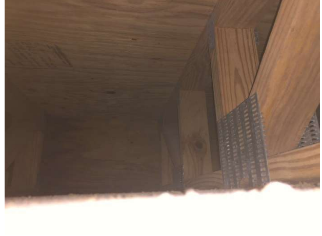
Staircase landing underside without wood rot or water intrusion evident
