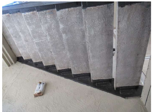
Underside of staircase
