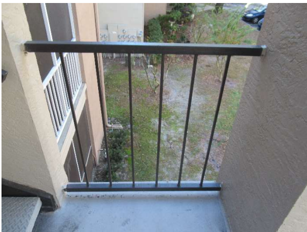
Railings at landings
