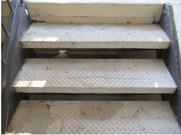
Tread cracks
